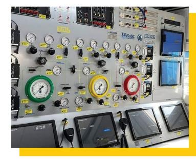
Full IMCA D023 DDC and DCC combo unit in 20ft DNV offshore container, that can convert even smaller vessels to the fully functional DSV. It is designed to support offshore diving operations up to the 50m depth and it can be used for up to 3 divers diving operations.
